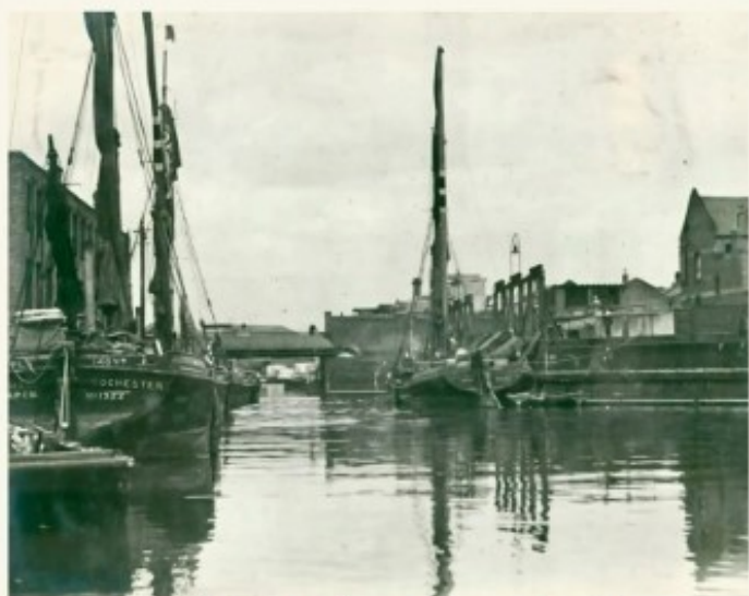
1930 Glengall Bridge from the west with Peckham branch on the right.
