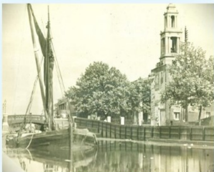
Surrey Canal and St George's Church Camberwell with Wells Way bridge 1934.
